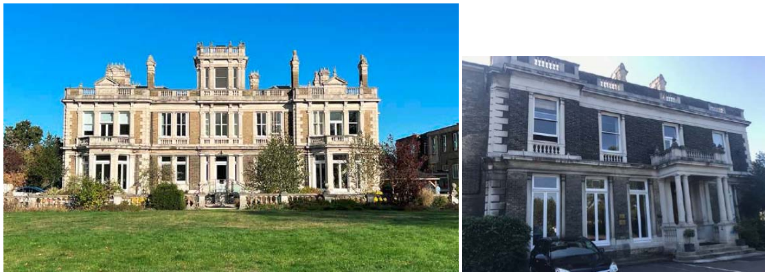
Figure 2: Photos of rear and side elevations
